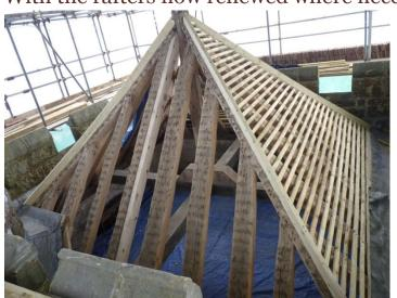
re-attached to the central post, the new batons are nailed on prior to re-tiling.
